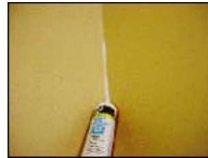
Caulking corners helps prevent future paint repairs.
